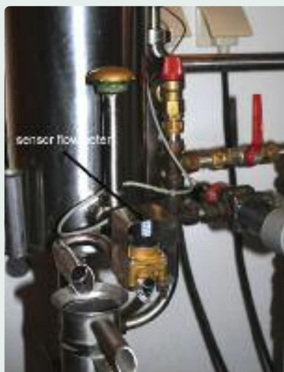
Right: Annotated photograph of the excise metering on the still. Below: The position of the sensor recording the hours of operation. Below centre: The flow sensor. Below right: The 'how often filled' sensor on top of the pot still.
